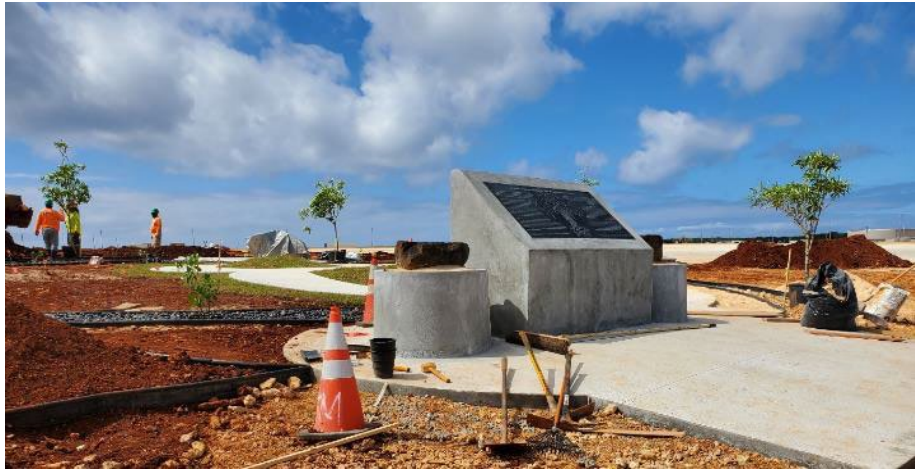
Progress Photo of Work: Monument with plaque, flanked by lusong, tree planting, the infinity path with grassy mounds and portions of the river rock oval are visible in the photo
